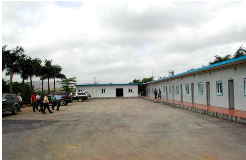
Figure 11 : Mine office complex and Crusher / Flotation Plant
