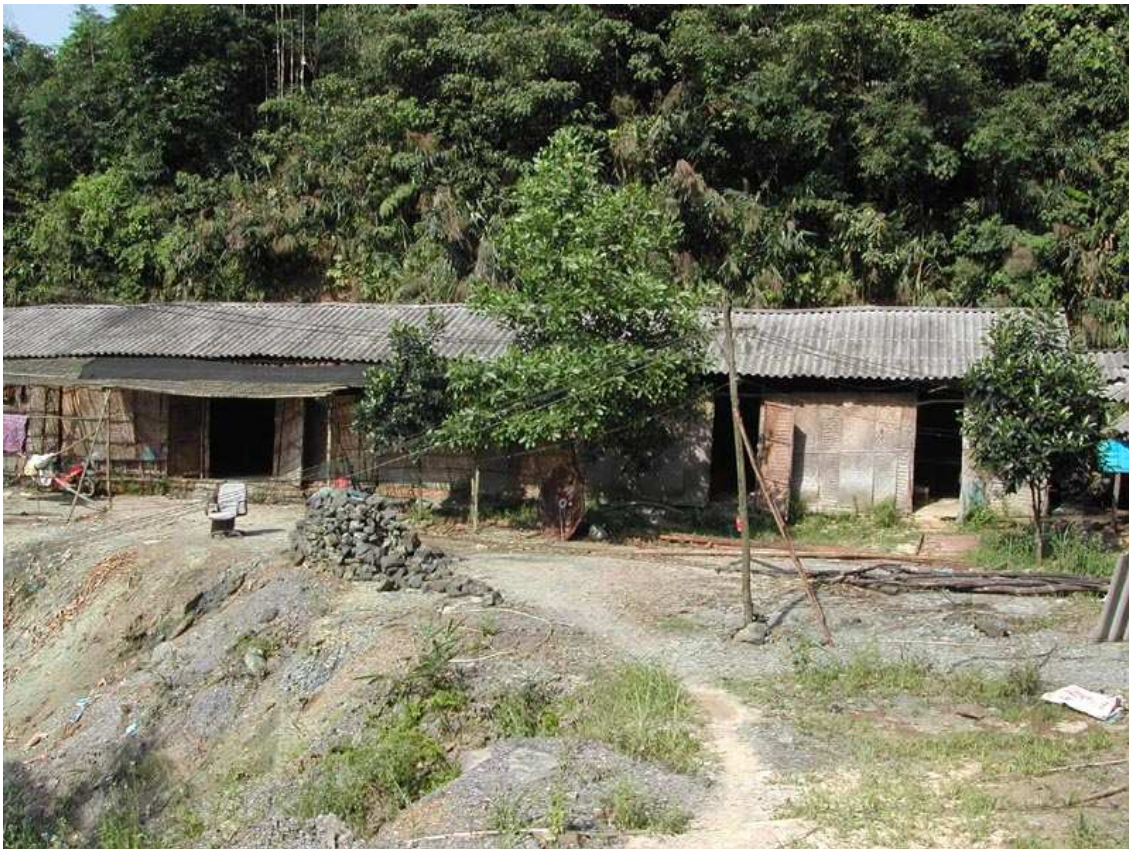
Figure 10 : Dong Quang III Mine : Mine Buildings and hand sorted heaps of high grade ore
