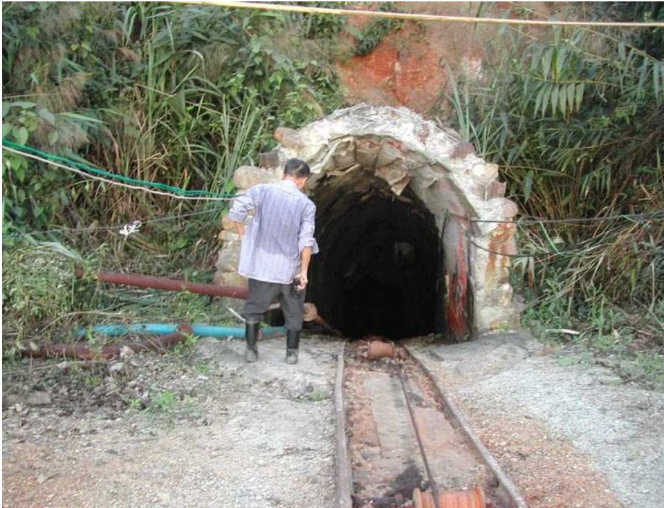
Figure 8b : Dong Mo Antimony Mine : View into mothballed decline
